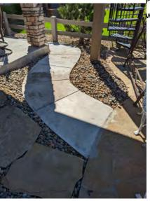
Pictures #5, 6 & 7 – These pictures show a more close up look of the grading on both properties and how they still slope towards the center after the sidewalk was completed. In the center photo, you can see how the neighbor's "old" sidewalk is tilted towards Norvel's property so that water would run off towards the center.
